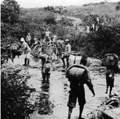
Figure 6.5: Lack of proper roads
